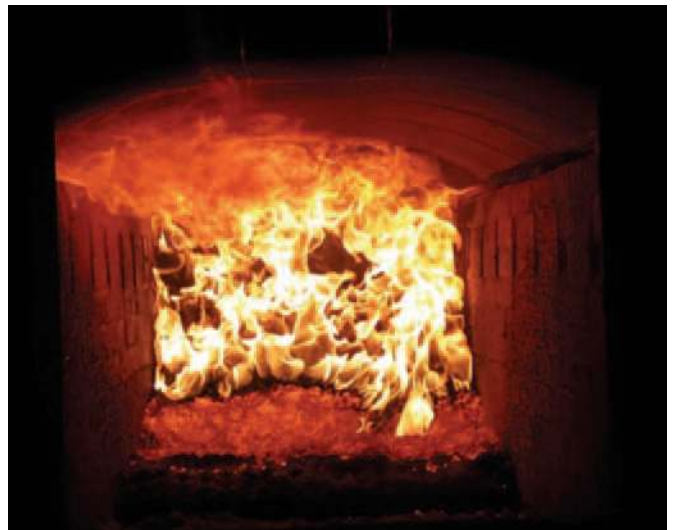
Figure 8 The step grate
